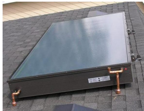
Roof mounted ICS or "Batch" collector
